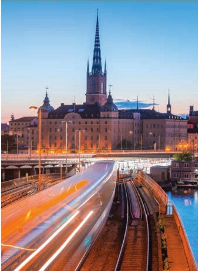
Vibration insulation of rail traffic reduces noise and creates good residential environments.
