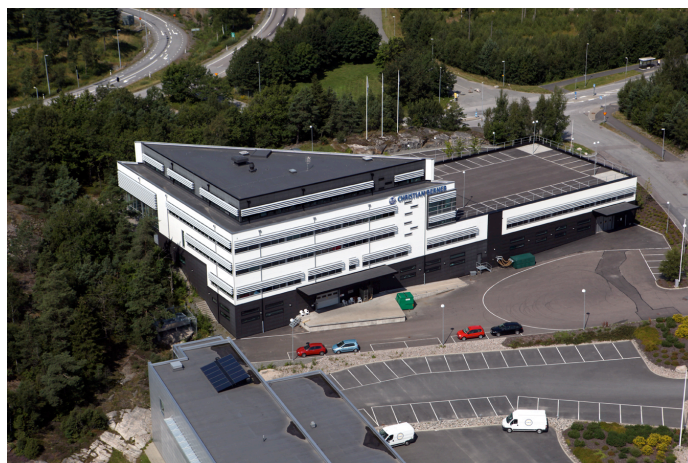
The property called Härryda Solsten 1:118 has a lettable area of approx. 5 000 square metres. Christian Berner Tech Trade AB has had its headquarters here since it was built 2006.
